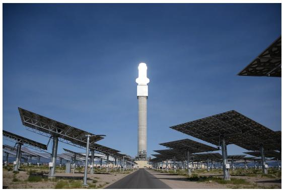
Large tracking mirrors, called heliostats, follow the sun throughout the day, reflecting and concentrating sunlight onto the top of Crescent Dunes' central tower. *Credit: SolarReserve* Molten salt's physical and thermal properties make it a
